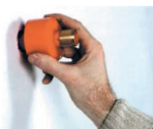
2. The rosette is inserted.
