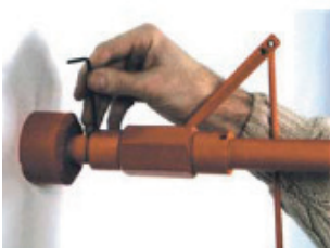
4. After alignment, the shower is fixed with Allen screws.
